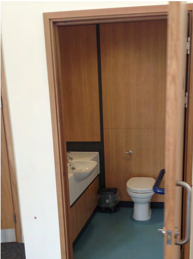
unisex paired cubicles, plus an accessible cubicle at Island of Portland Aldridge Community Academy, 2 - 18 in Portland, England
